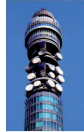
Telecom Tower – London, England
