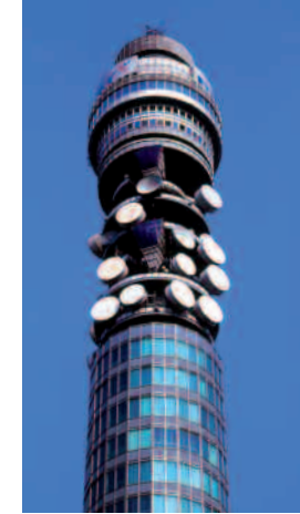
Telecom Tower – London, England
